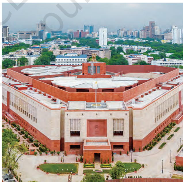
Fig. 6.3. The Parliament Building (Sansad Bhavan) in New Delhi was constructed to accommodate the growing needs including capacity, technology, sustainability and safety.
