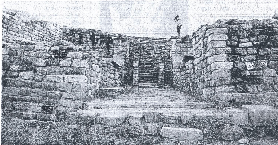
■ Civic lines: Dholavira in Gujarat has emerged as a major Harappan city remarkable for its town planning, architecture and water management system. ■ AFP
